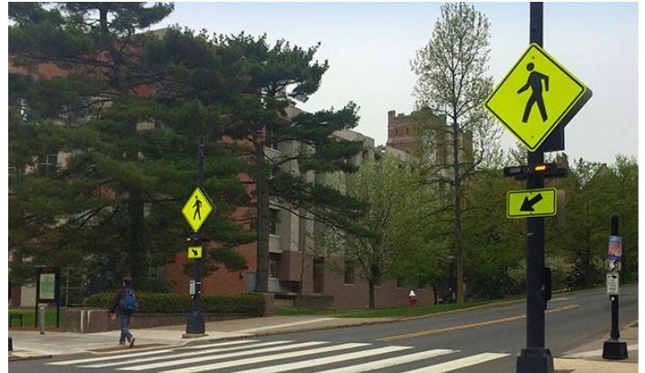
High-visibility crosswalk. (Source: FHWA)
